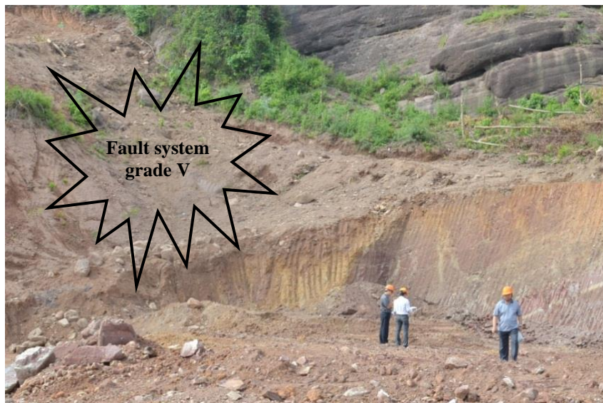
Fig. 3. Fault system grade V (main view from the Left Portal of the North Tunnel)
