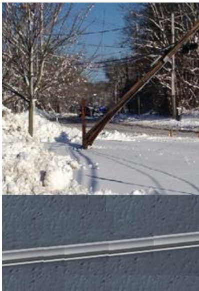
Figure 3 (left): Damage of overhead lines and reliability of underground cables from severe weather conditions.
