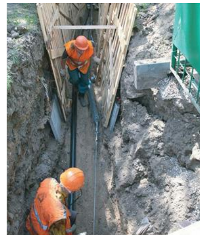
Figure 4 (right): Repair of underground cable. In figure 4 one can see repairs of underground cables.
