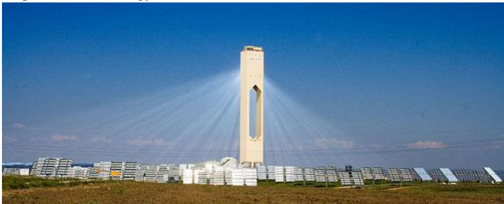
Picture 1, The 11MW PS10.
