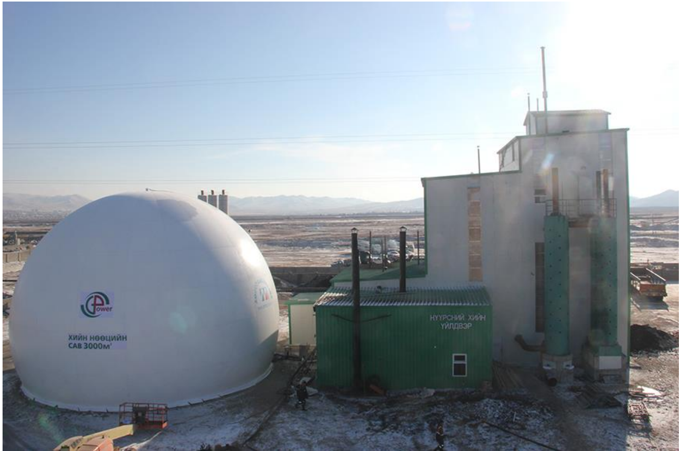
Picture 2. The plant has 1 set of gasifier, dust cyclone, air cooler, 2 sets of electric filters of coal tar, 2 sets of dryers, and 3000m 3 gas containers.
