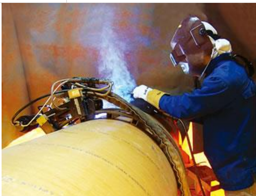
Figure 10 – Welding of pipe by PREMIARCTM DW-N625P and Magnatech machine. Photograph supplied, courtesy of Magnatech International B.V.
