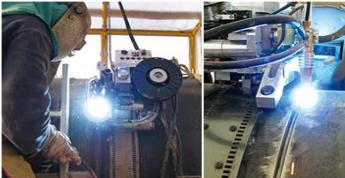
Figure 2: MAG welding by special girth welding machine. Photo courtesy of Pipeline Service S.r.l., Manufacturer of the Proteus FAP.
