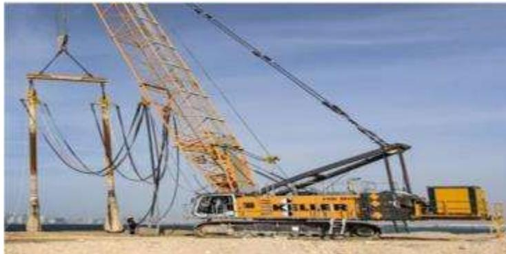
*Figure 3. Vibroflotation compaction*
