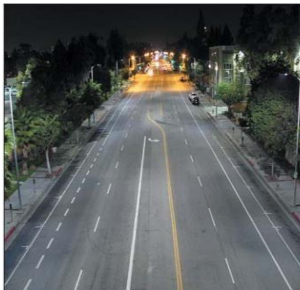
Figure 3 - Lighting Los Angeles
