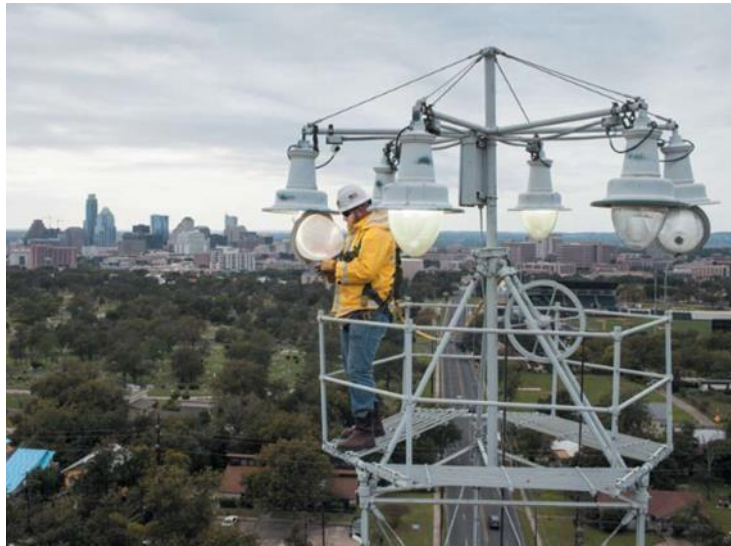
Figure 2 - maintenance of one of the lighting masts Austin
