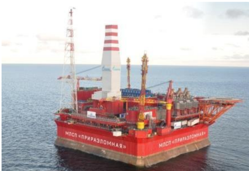
Fig. 3. The stationary ice-strengthened sea platform «Prirazlomnaya» in the Pechora Sea, Russia
