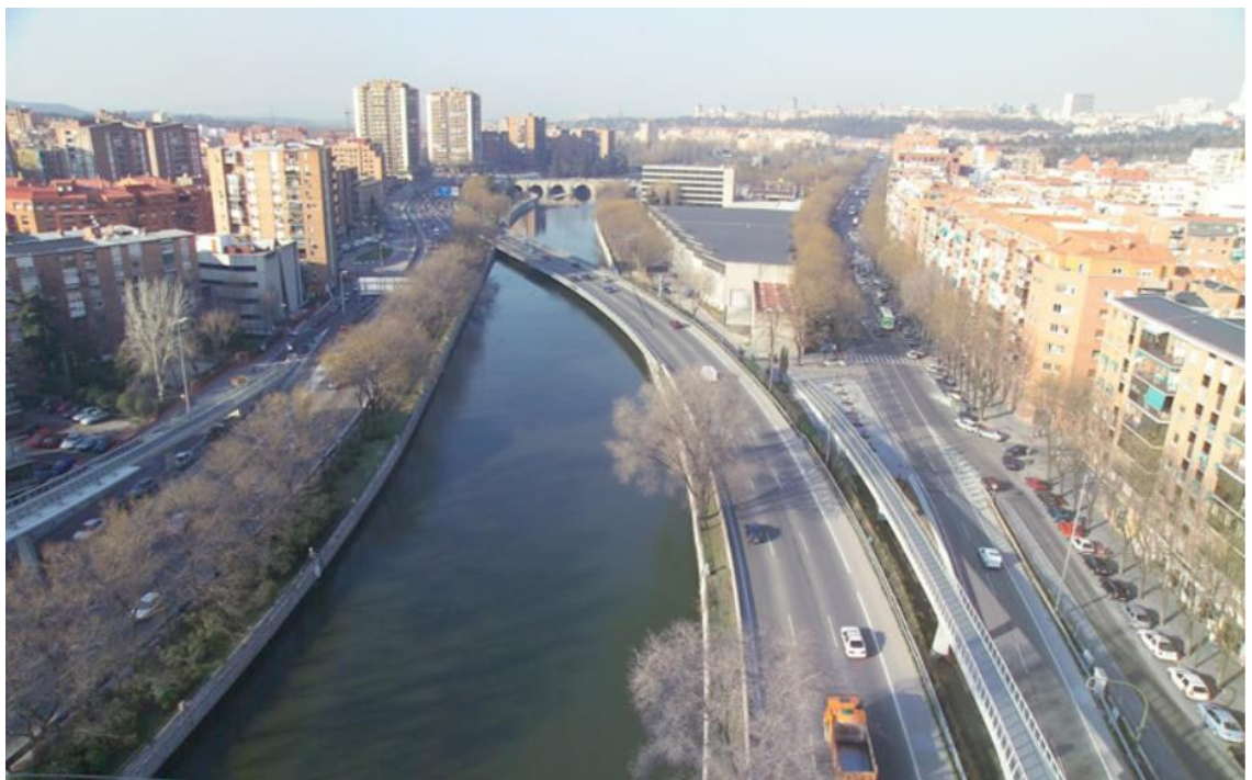
Figure 1. The highway before the renovation
