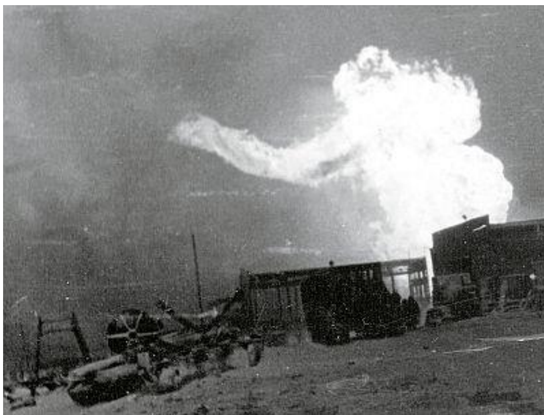
Figure 3. Gas pipeline accident in 1979
