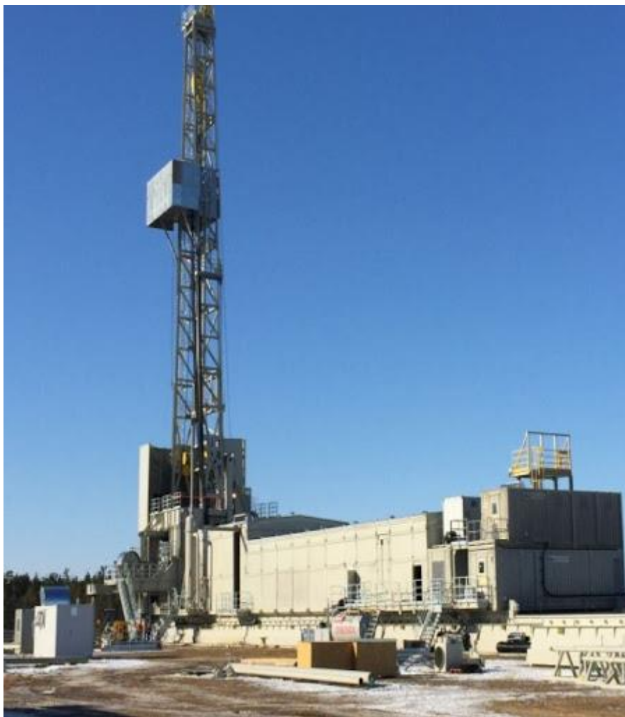
Picture 1 – Drilling rig Bentec HR–5000
