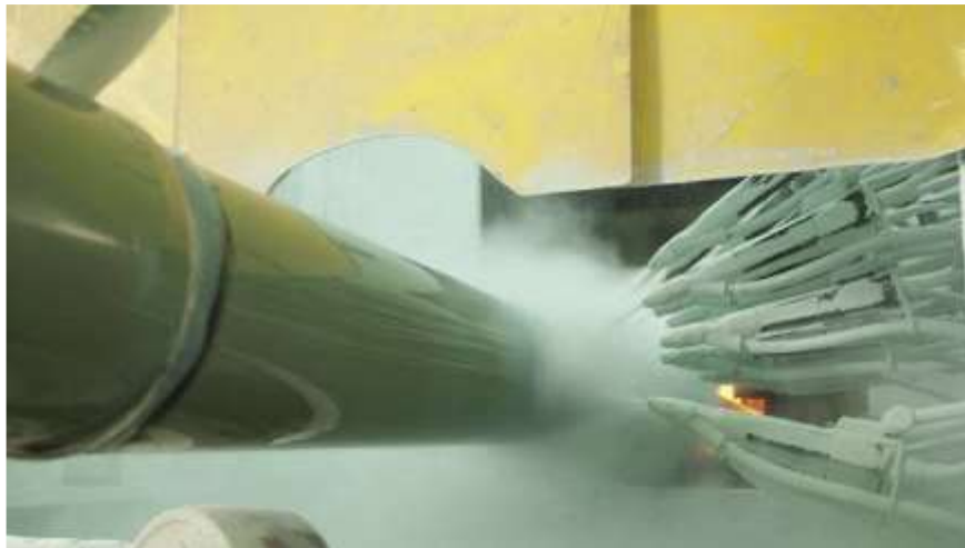
Figure 24.3 – Fusion-bonded epoxy powder application onto heated pipe [9].
