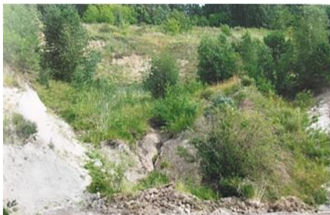
Figure 37 - Landslide Circus No. 1 on the site «Lagerny Garden», Tomsk [9]
