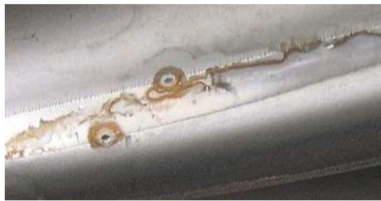
Fig. No. 14 - Surface failure of rotor coated with WC. Friction cuttings and initiation of formation of pits into the base metal due to coating thinning
