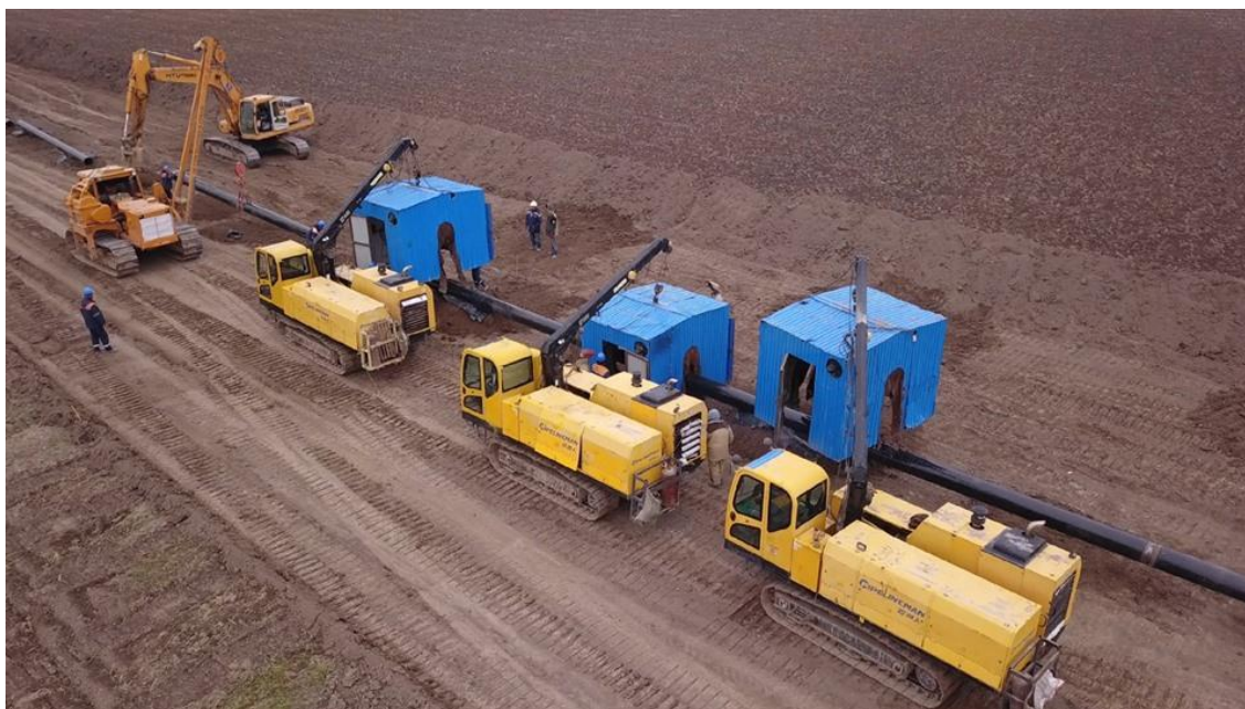
Picture 1. Construction of the main gas pipeline in the north of Kyrgyzstan
