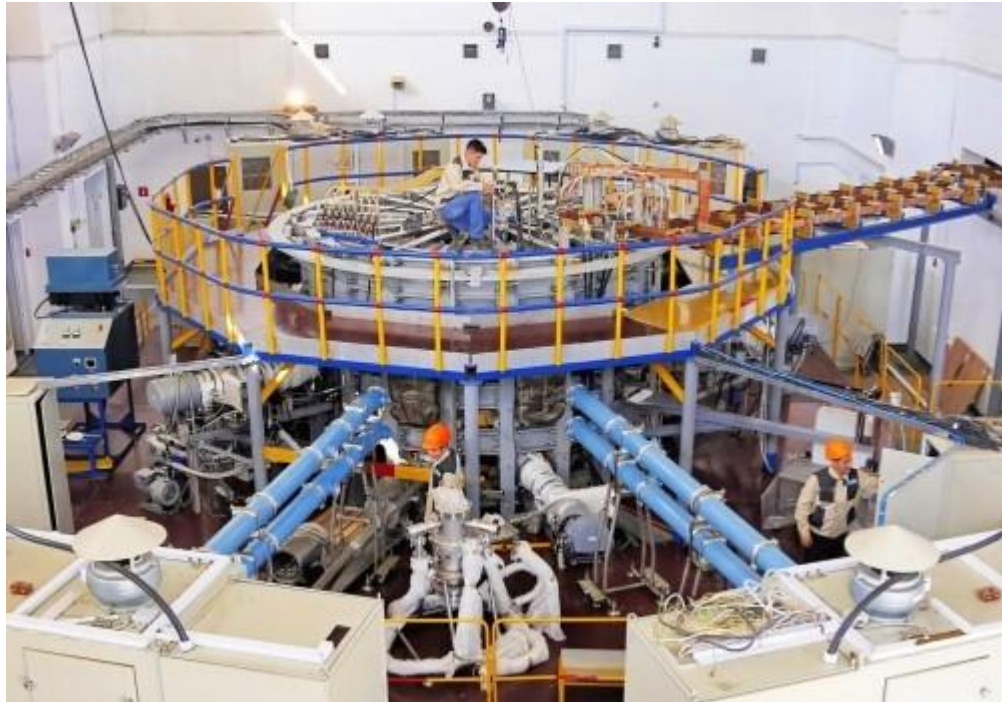
Figure 1 – General view of the KTM tokamak
