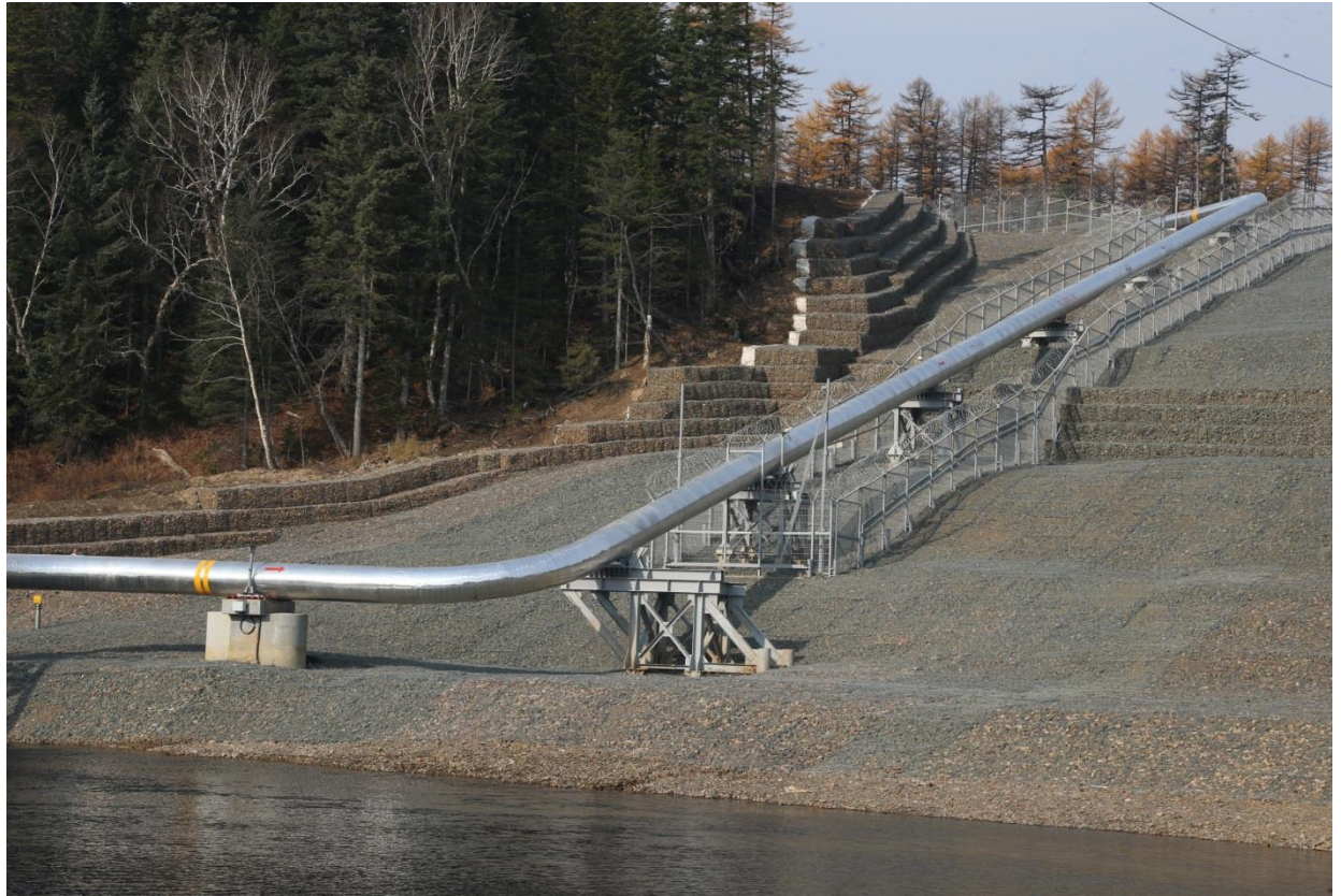
Pic. 2 – Bent branches used in above-ground routing
