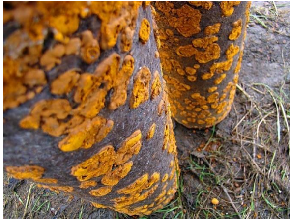
Picture 6 - example of biocorrosion
