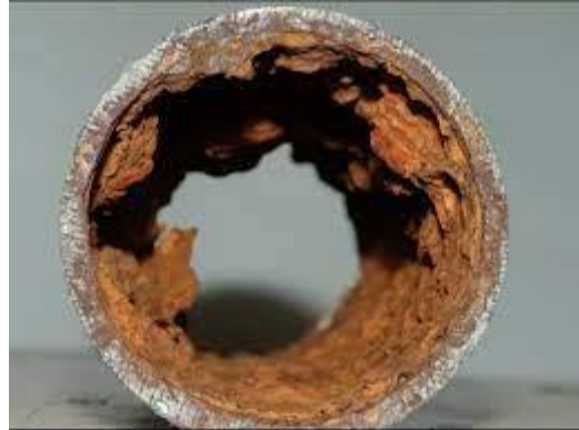
Picture 3 - example of gas corrosion
