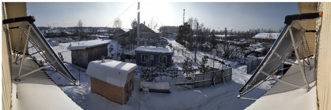
Figure 12. Panoramic photo of evacuated tube collectors with the shadow of the chimney of the gas boiler house.
