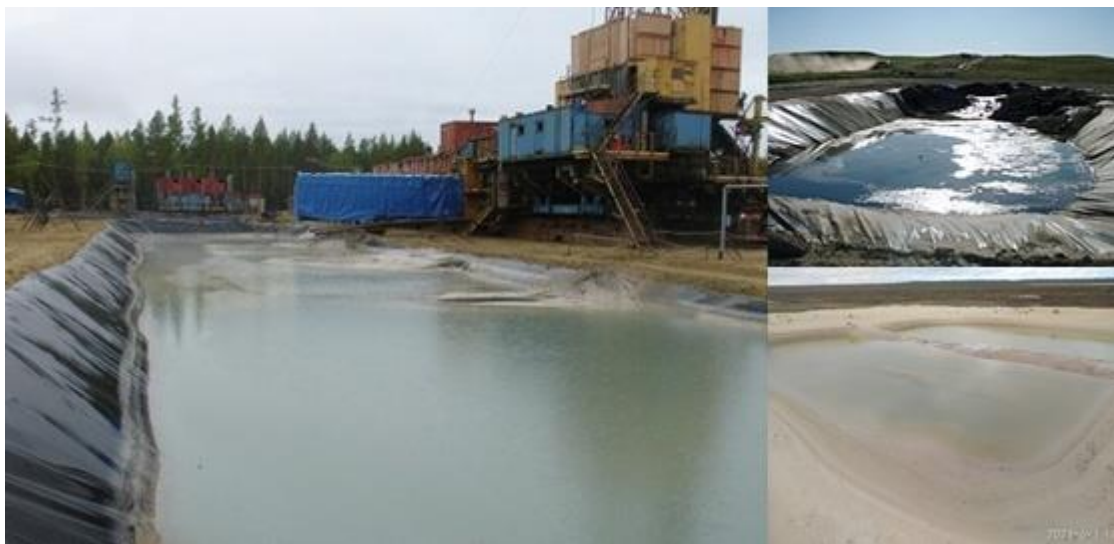
Figure 1 - View of the sludge pit (storage tank)
