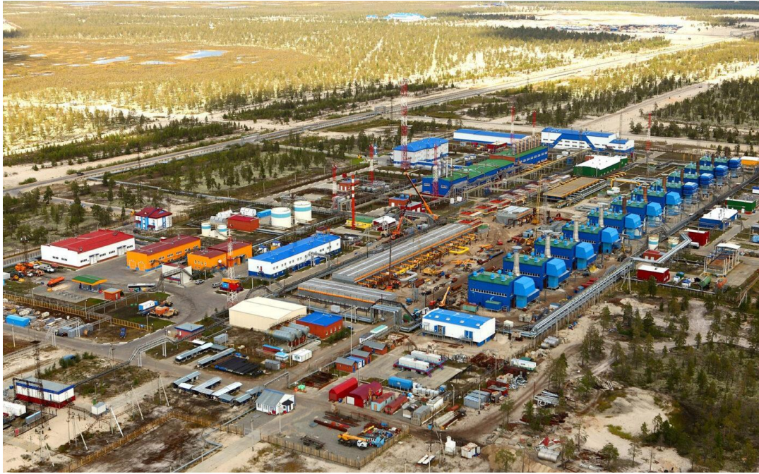
Figure 1 – Booster compressor station of the Vyingayakhinskoye gas field
