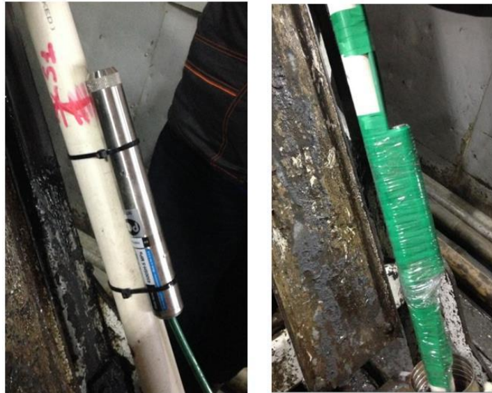
Figure 3-16: Installation of Geokon piezometer
