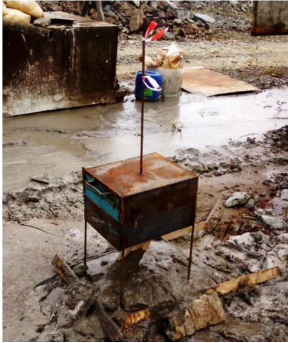
Figure 3-18: Protective box installed on top of the well
