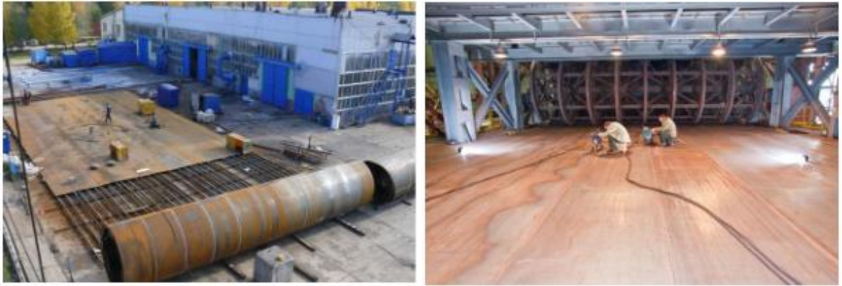
Figure 1 – Sheet metal tank wall assembly in open and closed site conditions
