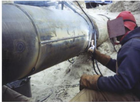
Figure 9 – Installation of Type B full-encirclement repair sleeve
