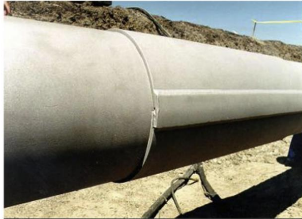
Figure 8 – Type A encirclement repair sleeve with fillet-welded overlapping side strips
