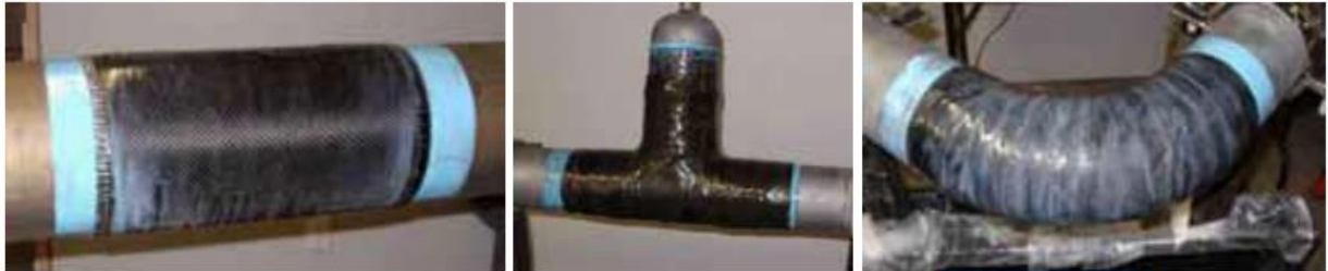
Figure 3 – Structures repaired by the Black Diamond system
