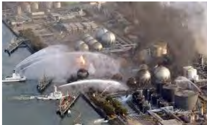
Fig. 1. Using fire engines to remove the decay heat at Fukushima Daiichi
