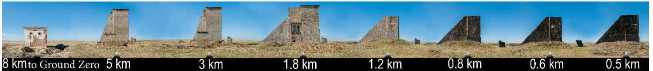
Figure 5 – The way instrumental structures currently look southeastward
