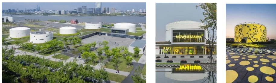
Fig. 2. Shanghai Oil Tank Art Center, China
