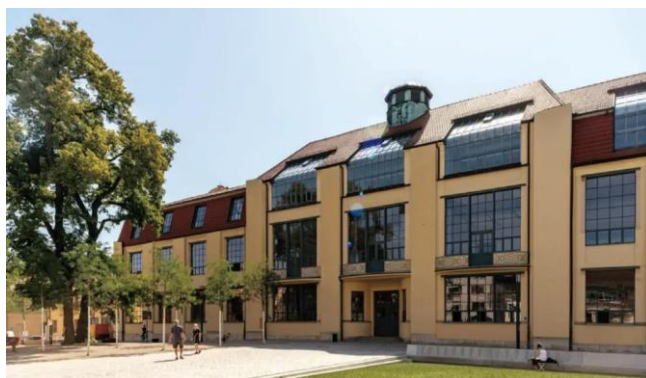
Fig. 2. Teaching building of Bauhaus University in Weimar, designed by Henry van de Velde, the first building to use glass curtain wall as facade
