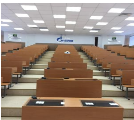
Figure 3.1.5–Installation of energy-efficient light fixtures in the room. No. 204.MB
