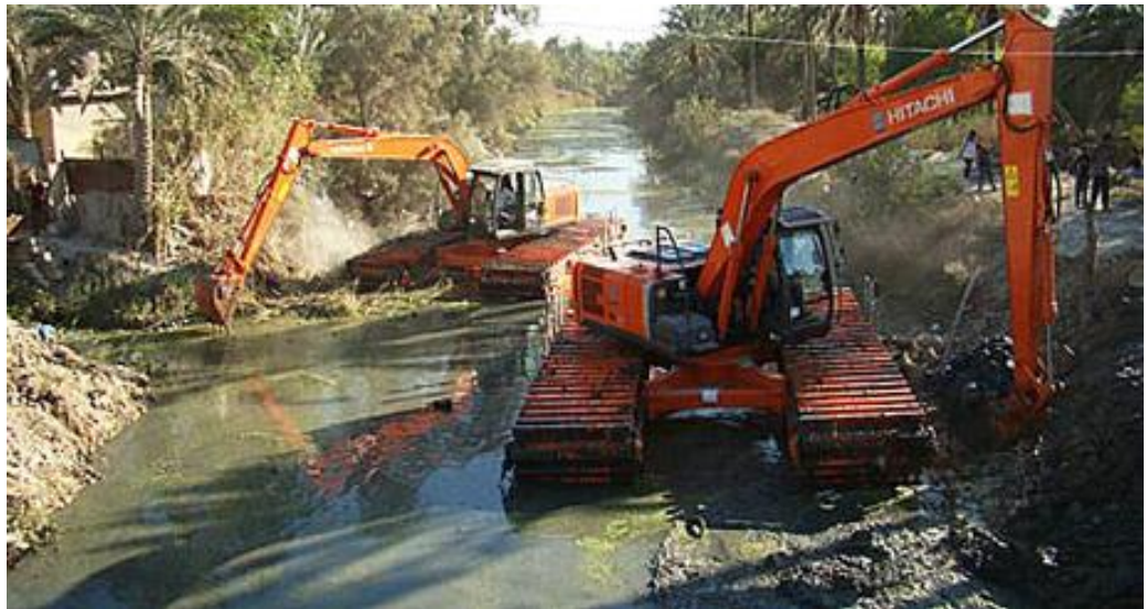
Figure 2.7 Amphibious Excavator Hitachi 200 MA
