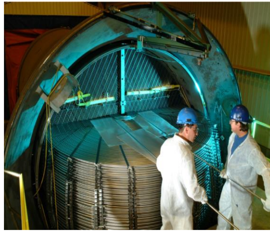
Figure 1.4 - Steam generator tube installation
