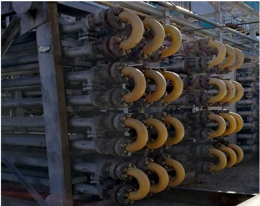
Pic. 7 Refrigerator 1 stage compressor 2 stage.
