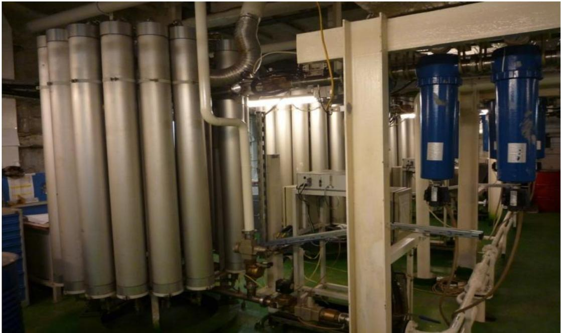
Figure 9 - Membrane gas separation installation
