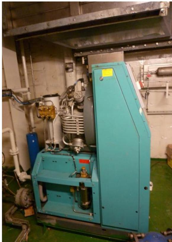
Figure 12 - Booster compressor GIB 15.3-11-5
