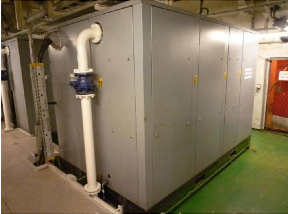
Figure 11 - Atlas Copco GA-250-13 Compressor
