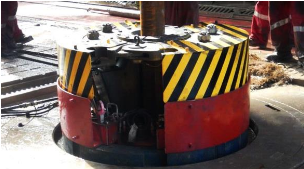
Figure 54 – Descent of casing strings
