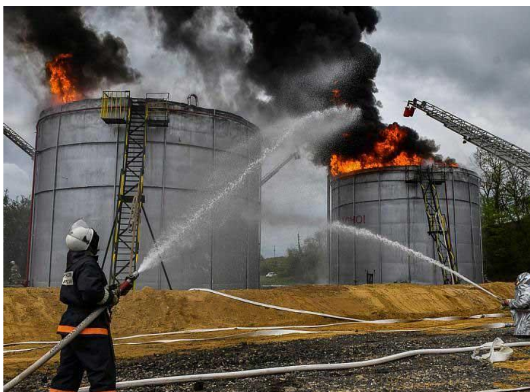
Figure 13 – Storage tank accidents
